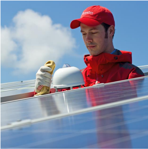
Figure 1 maintenance of SR20 secondary standard pyranometer with VU01 ventilation unit in PV system performance monitoring, measuring plane of array irradiance
