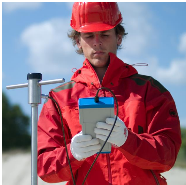
Figure 1 Soil thermal route survey with FTN02 including CRU02 control and readout unit
